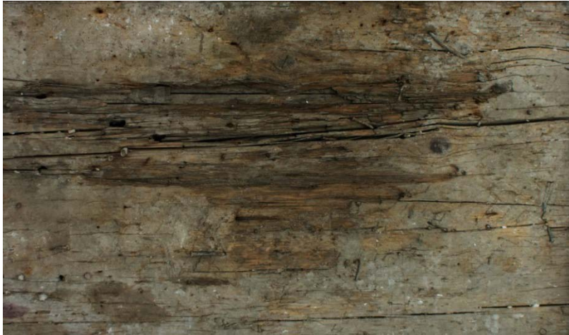
Fig.10. Wood decaying under the influence of water, clay, plaster
